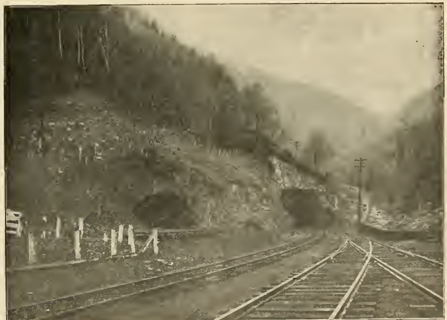
WEST PORTAL OF THE HOOSAC TUNNEL, SHOWING ABANDONED ENTRANCE.
